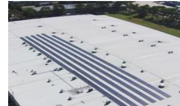
On site solar across 5 sites – 7,547 MWh
